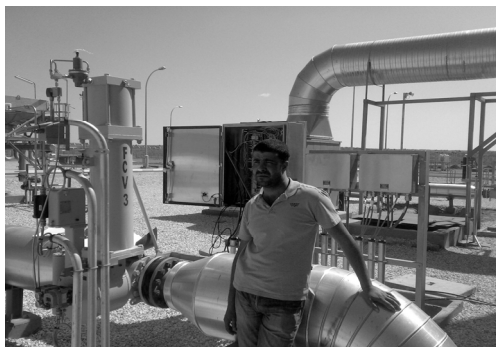
Figure 1.c. Anti-surge valve used in compression system
